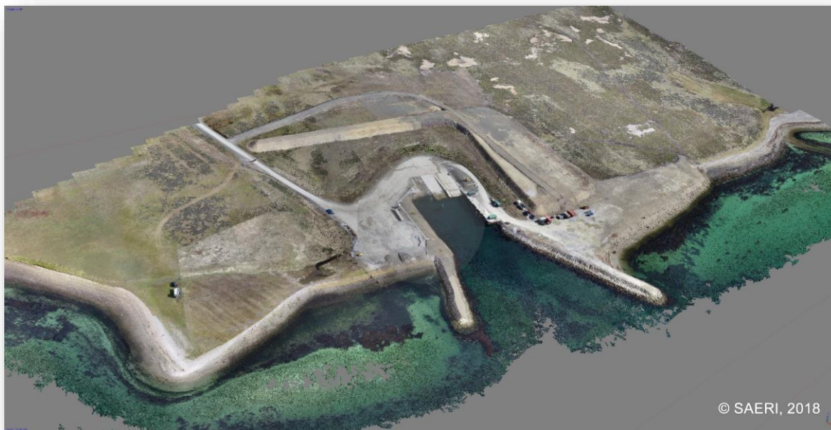
Figure 4.1: An example of the type of imagery/3D models collected/developed from drone mapping missions – Newhaven ferry terminal and surrounding area.
